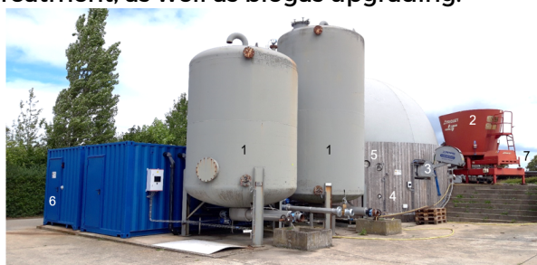
Overview of the biogas pilot plant (Pocket digester (31 kWel)) at Inagro: (1) Silage tanks to store and feed liquid pig slurry; (2) Trioliet screw press to feed the faecal fraction of pig manure; (3) Mixing system; (4) Reactor; (5) Air injection for biological desulphurization; (6) CHP; (7) Partially covered trench silos for the storage of the faecal fraction of pig manure.
